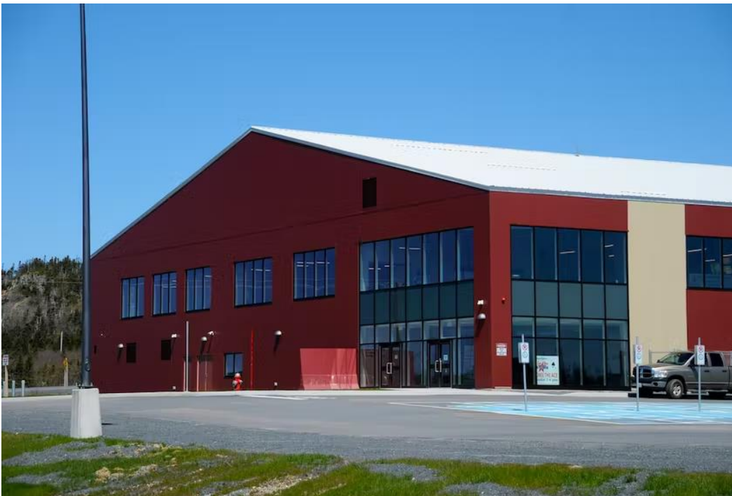
Figure 1: Danny Cleary Harbour Grace Community Centre
